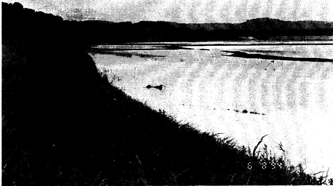
Figure 1. Excellent vegetative cover on interior slope of dike in area no. 2. Note small trees growing on interior.
