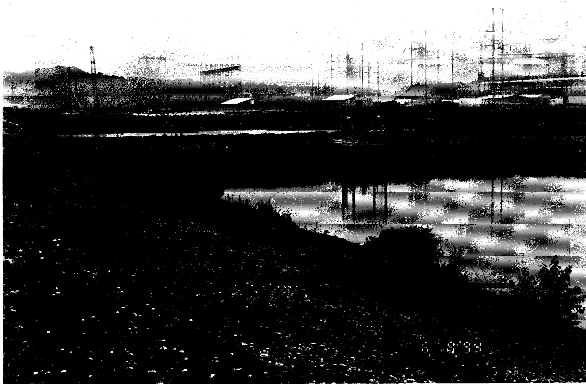
Figure 6. Chemical treatment pond with excellent riprap cover on the dike slopes. Coal yard drainage basin is in background with good vegetative cover on the dike slopes
